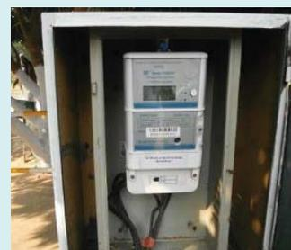
Figure: Prepaid smartcard operated machine
