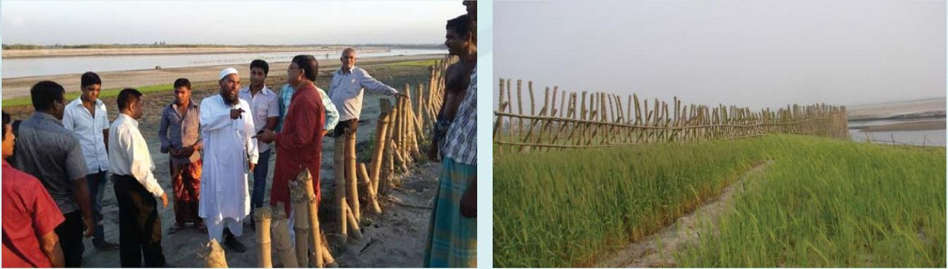
Figure 4(a): River bank sedimentation (3.5 m) instead of erosion; Figure 4(b): Crop production in place of river bank erosion [The officials of the BCCTF are visiting the performance of the bamboo bandalling structures constructed in the Old Brahmaputra River near North Sirajabad of Islampur Upazila under Jamalpur District The BCCTF officials are visiting the project site (left) and bumper wheat crop cultivated in the bank protected area (right)]
