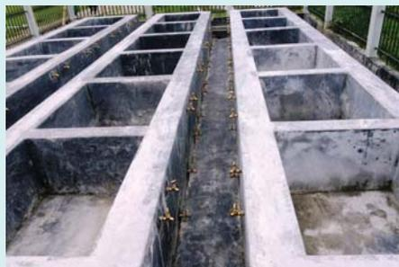
Figure 1: View of Lysimeter after completion of construction (before filling soil)
